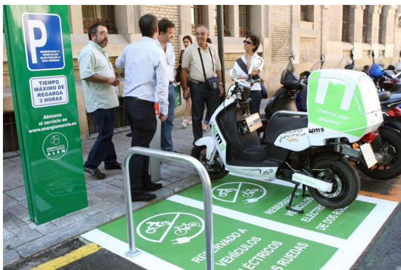
Image 3: Charging point for two-wheeled electric vehicles in Paseo Alfonso X
